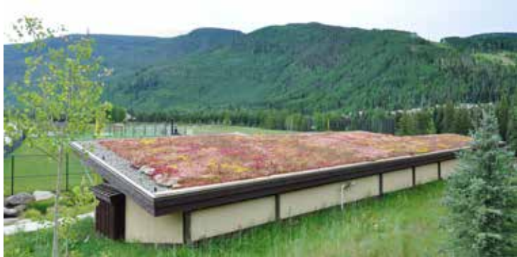
Green Roof at West Maintenance Facility, Vail, Colorado
