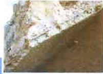
Plaster aqueduct interior
