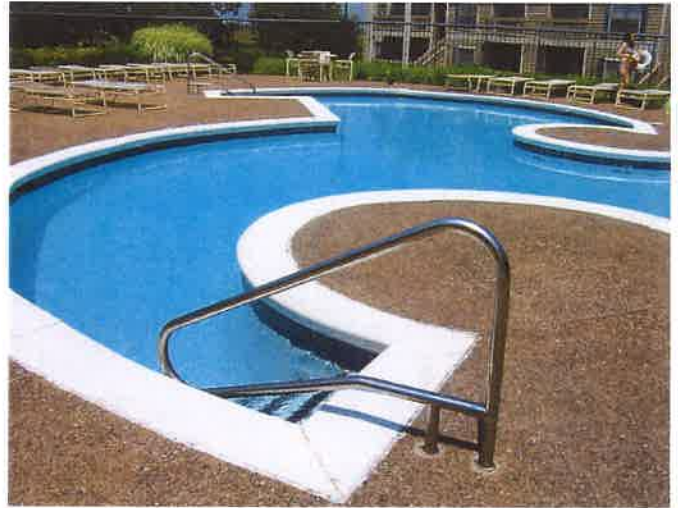
Pool re-plastered by Mid-America Pool Renovation, Inc.
