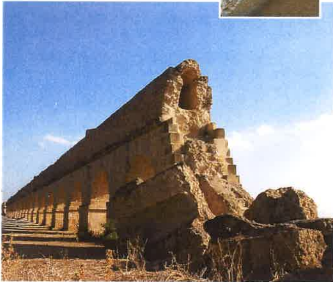
Roman aqueduct to carry water
