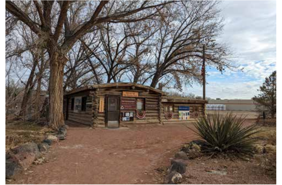
The Fort Uncompahgre Interpretive Site building.
