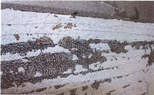
Pool Surface After Hydro-Blasting
