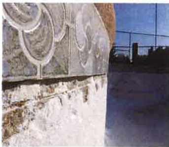
Saw-cut and chip below tile
