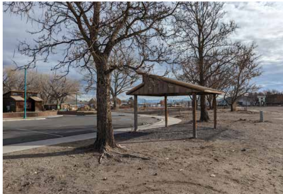
The existing timber shelter on the north side of the site. The existing parking lot is to the north of the shelter.
