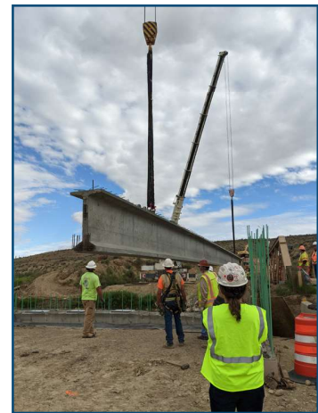
Girder Placement at CR 73
