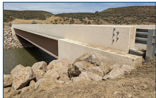
Completed Bridge at CR 73
