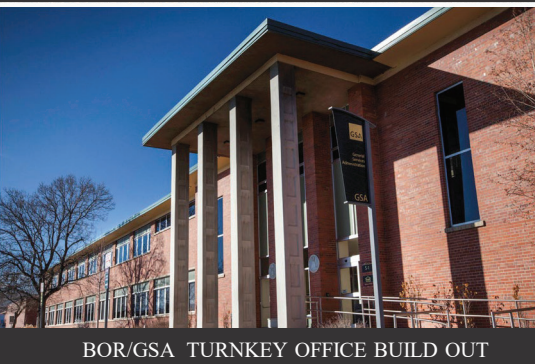
DENVER FEDERAL CENTER MULTI PROJECT AWARD
