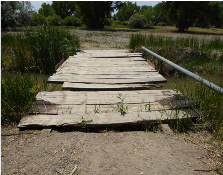
Existing Bridge over Canal
