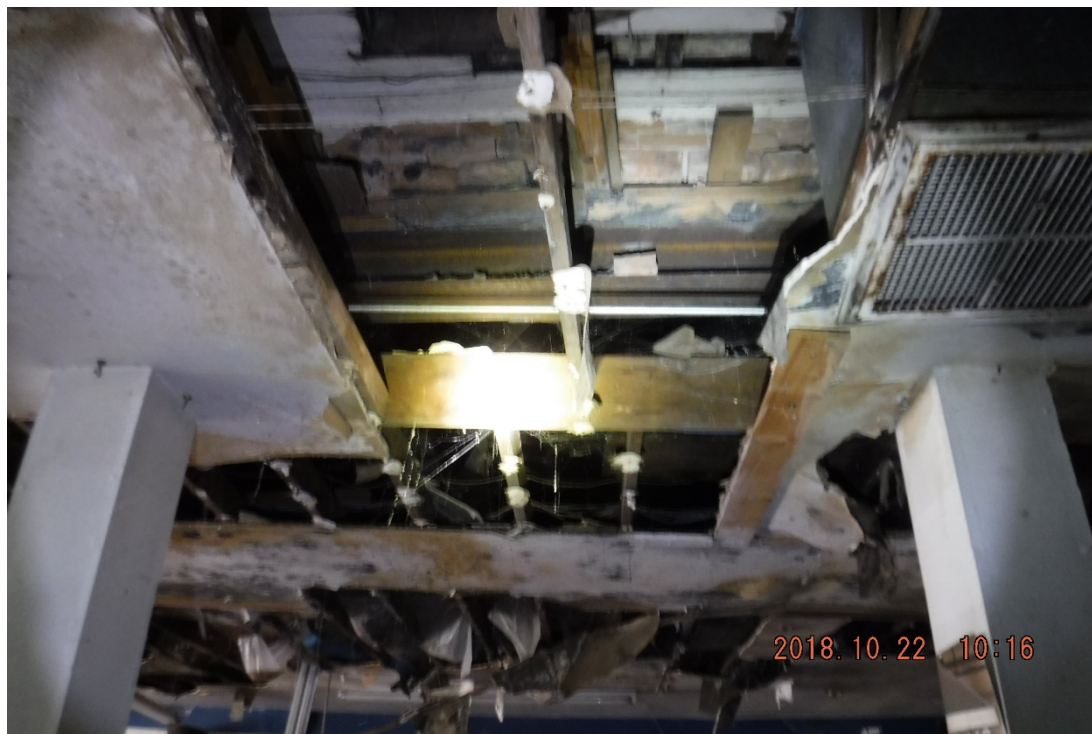
Photo 6 - Steel Beam A & Wood Framing
