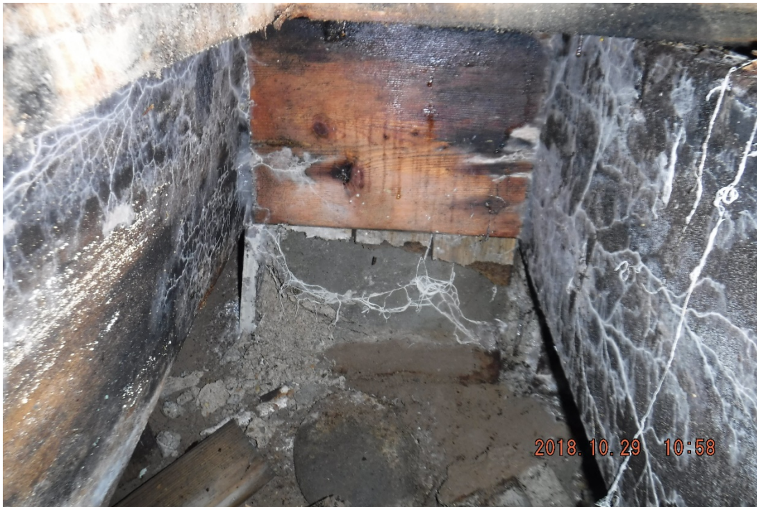
Photo 8 - Concrete Footing Below Beam A
