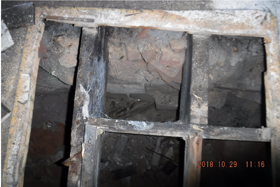
Photo 9 - Stone Foundation Below Beam B
