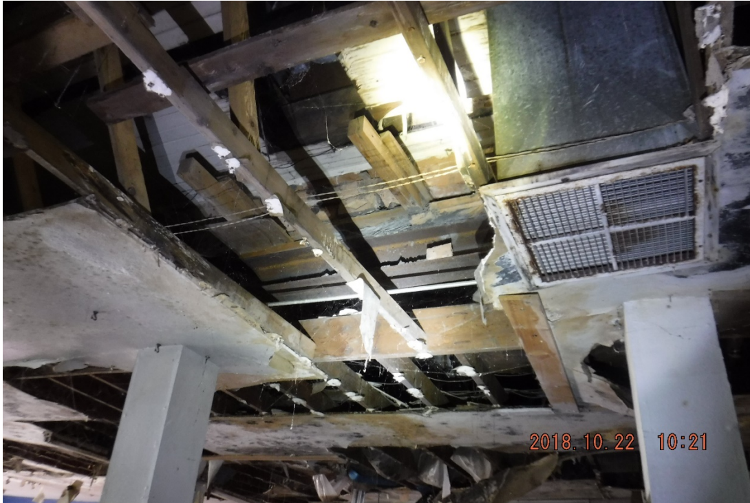
Photo 7 - Steel Beam B & Wood Framing
