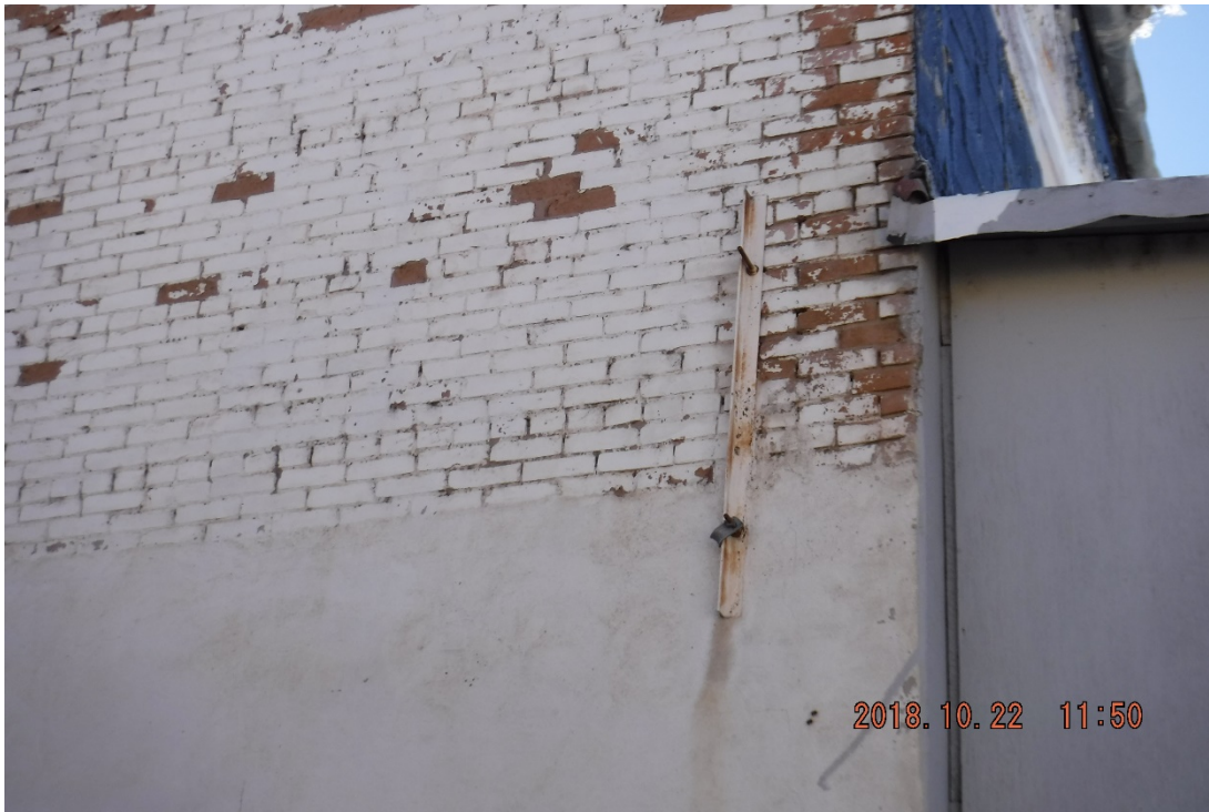
Photo 15 - Tension Ties Intersection Gridline 1 & C
