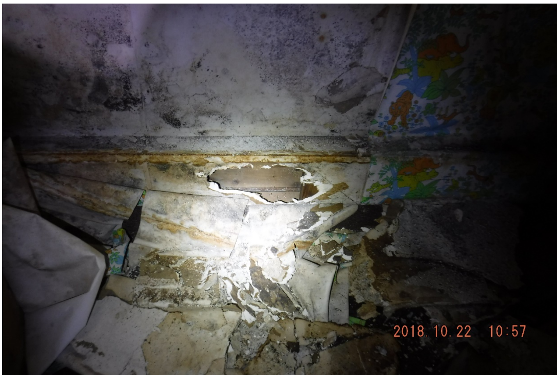
Photo 16 - Tension Tie In Wall Along Gridline C
